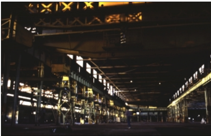
The gantry crane from the former Canron Building will be re-erected in a public space in SEFC to commemorate the shipbuilding heritage of the site
