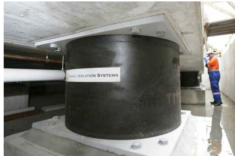
Technologies such as piling, ground densification base isolation (pictured above) will help improve the resilience of structures on site. (Source: civildigital.com )
