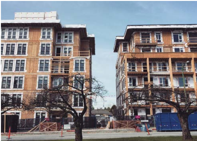
Multi-family timber frame construction, Cambie Street (Source: Aaron Lao)
