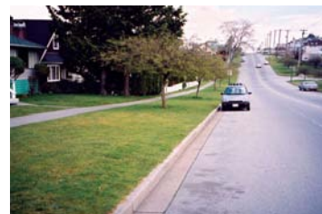
Curb and gutter
