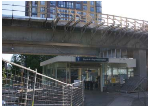
Ongoing station upgrades
