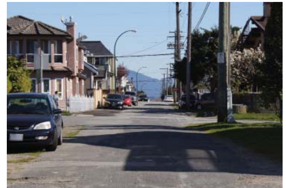
Missing sidewalks along McHardy Street
