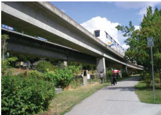
Elevated guideway above a community garden
