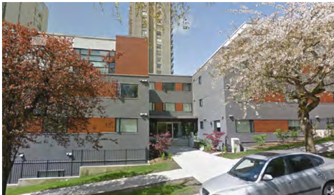
Figure 5.21: Examples of alphabet buildings with entry courtyards
