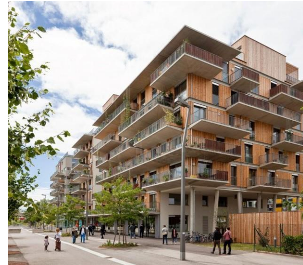
Figure 11.1 - Generous liveable balconies
