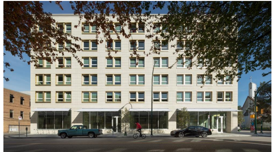
Figure 19.3 - Brixton Flats: One of Vancouver's first multi-unit buildings to meet the Passive House standard
