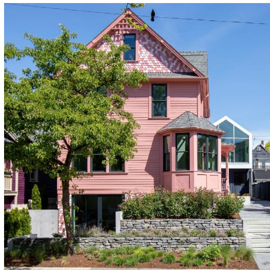
Figure 11.24 - Multiplex heritage restoration. Photo credit: MA+HG Architects
