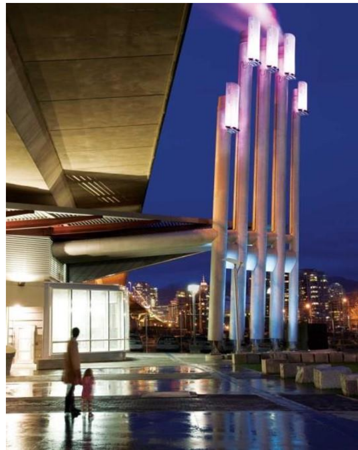
Figure 19.1 - Southeast False Creek NEU under the Cambie Bridge
