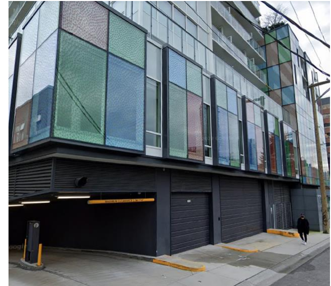
Figure 11.21 - Underground parkade entrance integrated into building architecture
