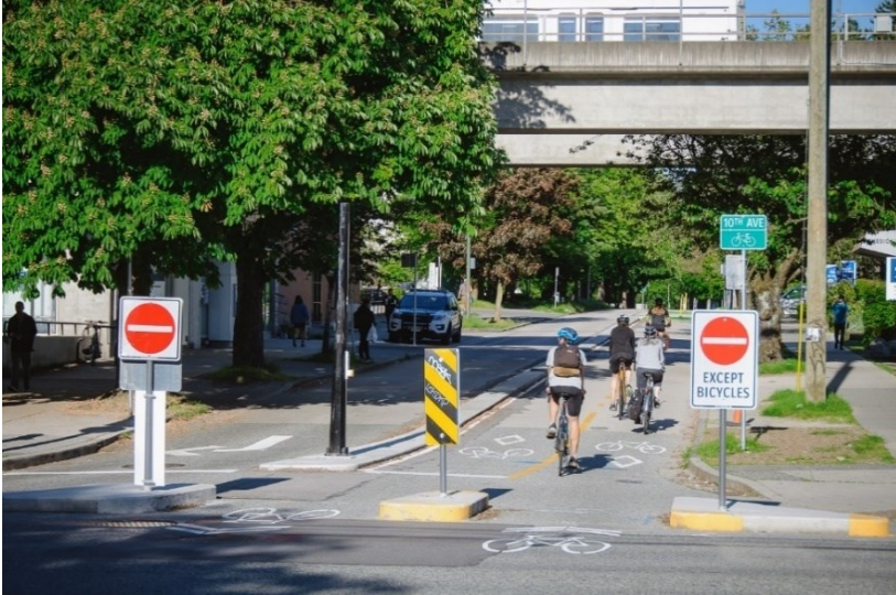
Caption: Bi-directional active travel lanes on 10 th Avenue at Commercial Drive with one-way vehicle access. (credit: Dylan Passmore)
