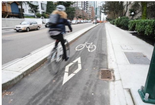
Caption: Uni-directional active travel lane on Pacific St with two-way vehicle access and no curbside uses (credit: Rod Preston)
