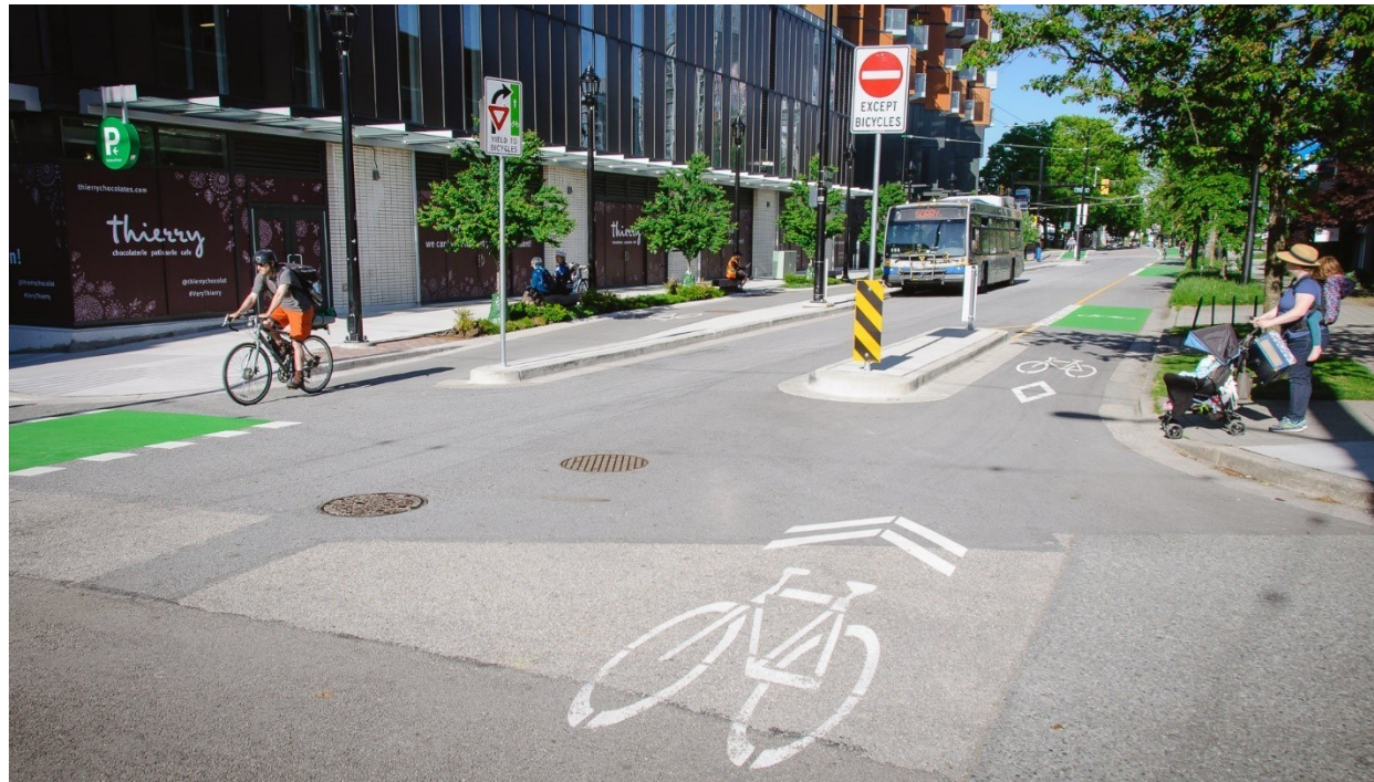
Caption: Uni-directional active travel lanes on 10 th Avenue between Watson Street and Kingsway make it safer and more comfortable for people rolling and cycling on streets where there are higher traffic volumes including from transit vehicles. (photo credit: Dylan Passmore)
