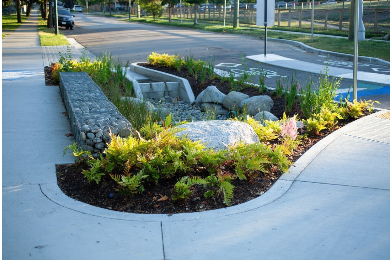
Figure 63: Sunset Park green infrastructure
