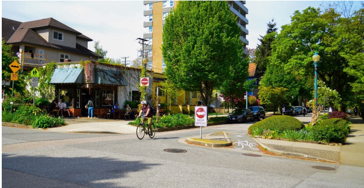
Caption: A partial closure created through road space reallocation at 10th Avenue and Quebec Street limits westbound vehicle access to provide a safe and comfortable environment for people walking, rolling, and cycling. Curb bulges at the intersection provide additional opportunities for planting and placemaking and on-street parking has been provided on one side of the street. (photo credit: Steve Chou)
