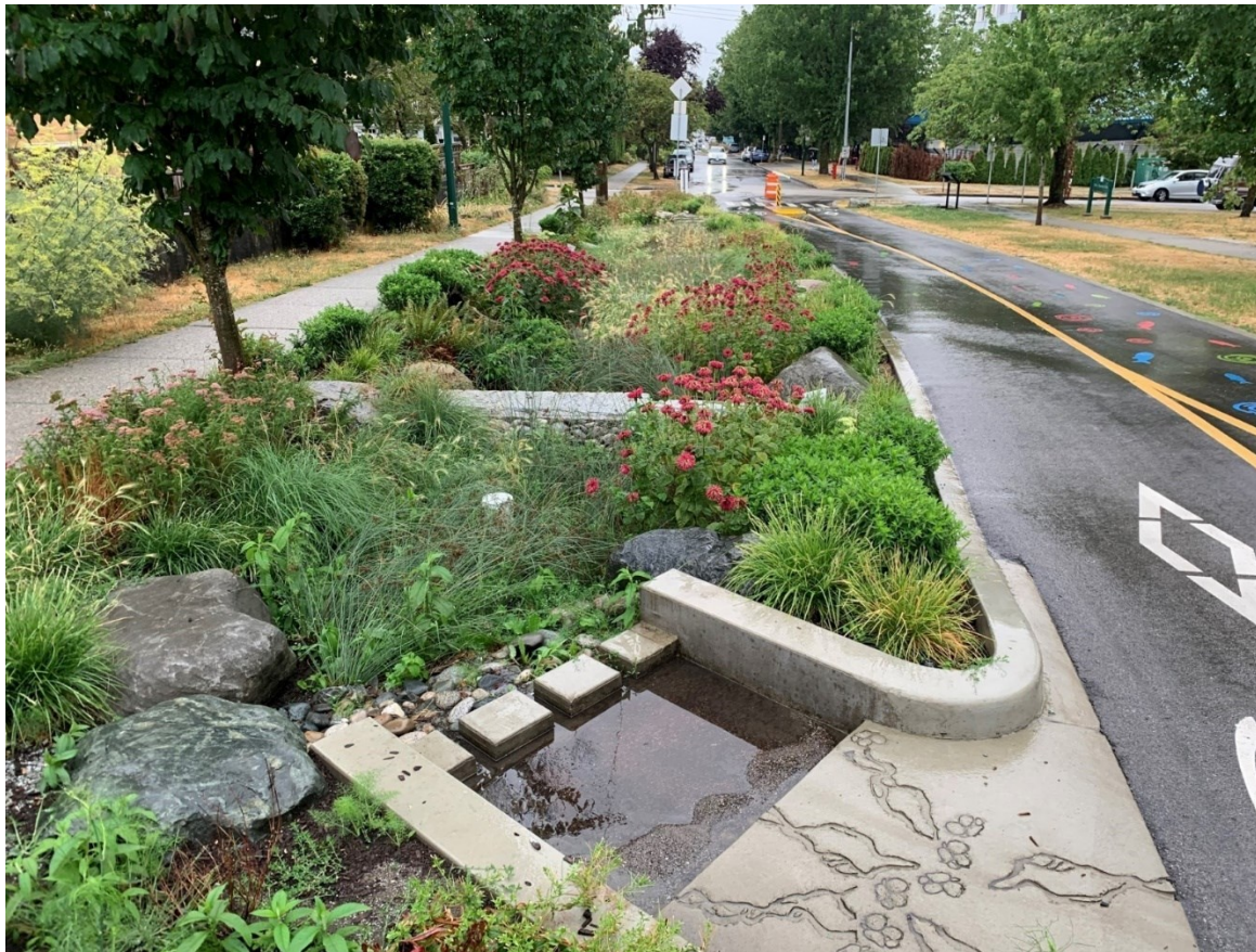
Figure 61: Woodland Drive and East 2 nd Avenue bioswale
