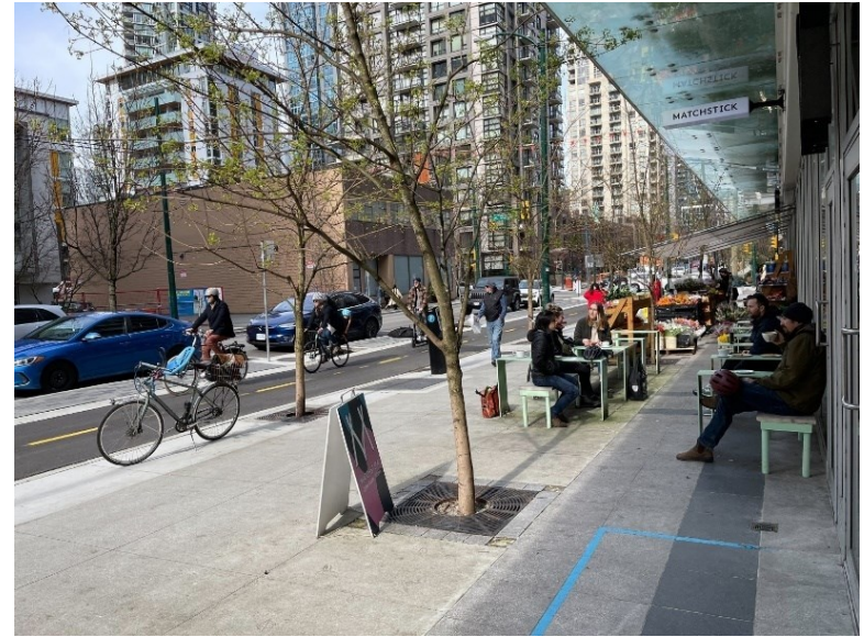
Caption: Bi-directional bike lane on a one-way street on Richards Street with a parking buffer and wide sidewalks to allow for many uses on the street. (photo credit: Paul Krueger)
