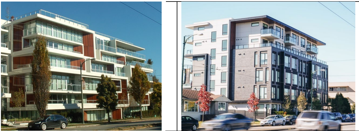
Figure 7: Varied rooflines on apartments
