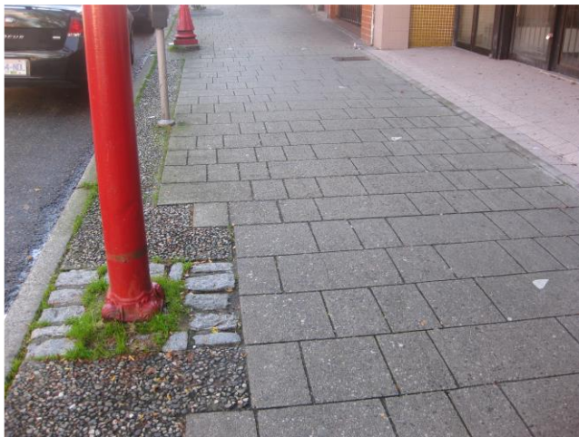
Figure 11. Sidewalk paving pattern and granite cobblestones detail
