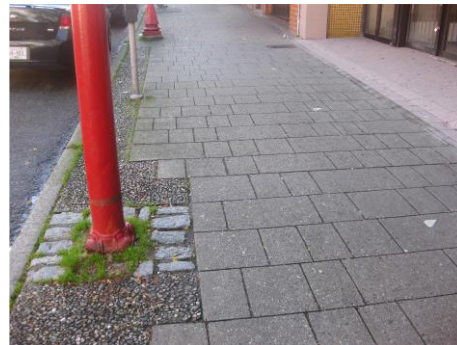
Figure 22. Sidewalk paving pattern and granite cobblestones detail
