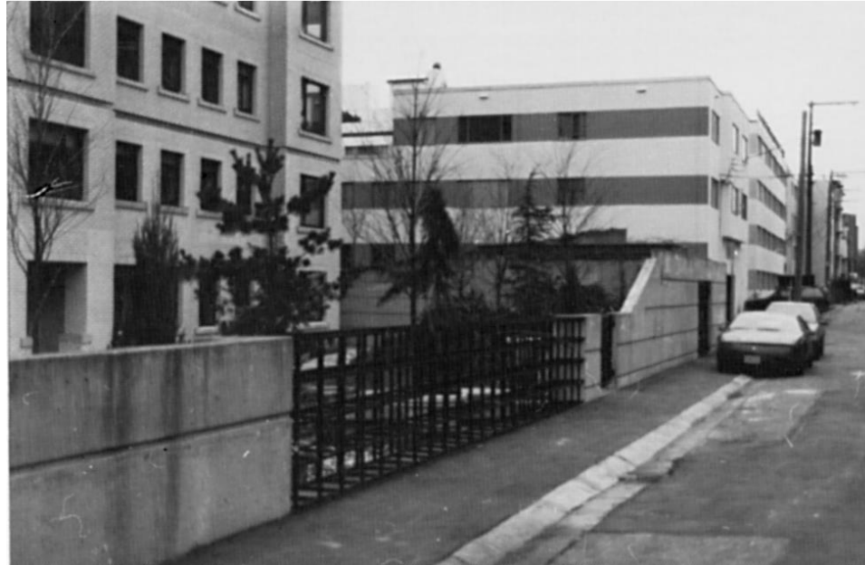
Figure 17. Attractive Exterior Wall
