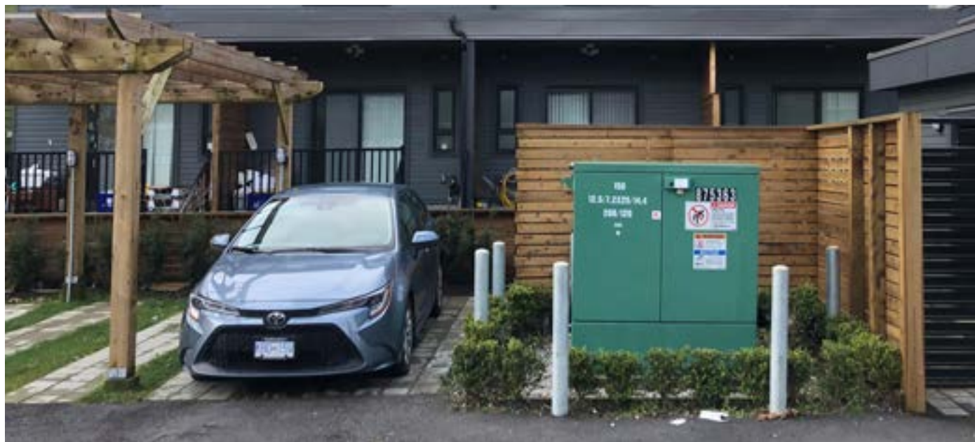
Pad mounted transformer. Credit: City of Vancouver
