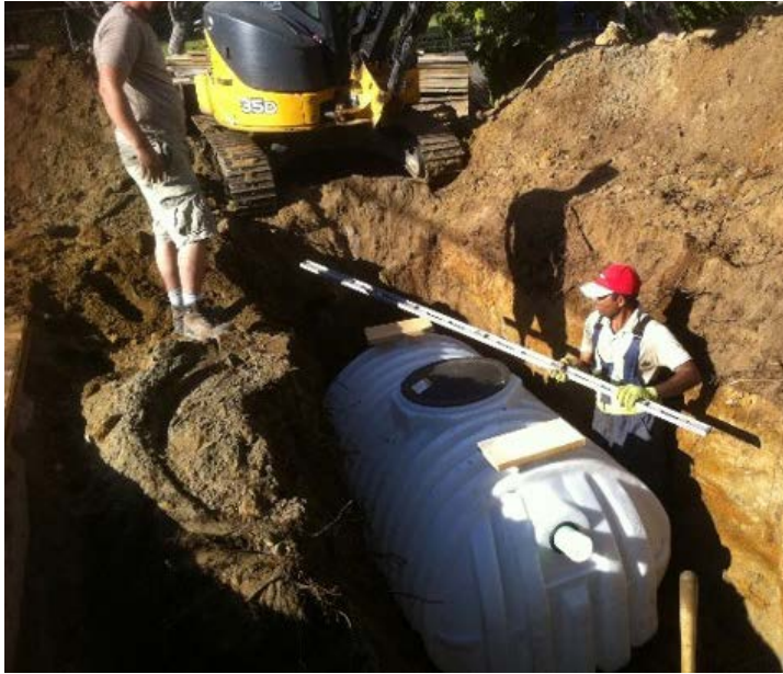
Detention tank installation. Credit: Lanefab Design/Build
