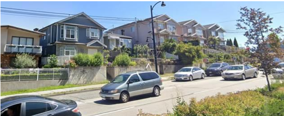
Figure 2. Example of existing grades higher than City building grades
