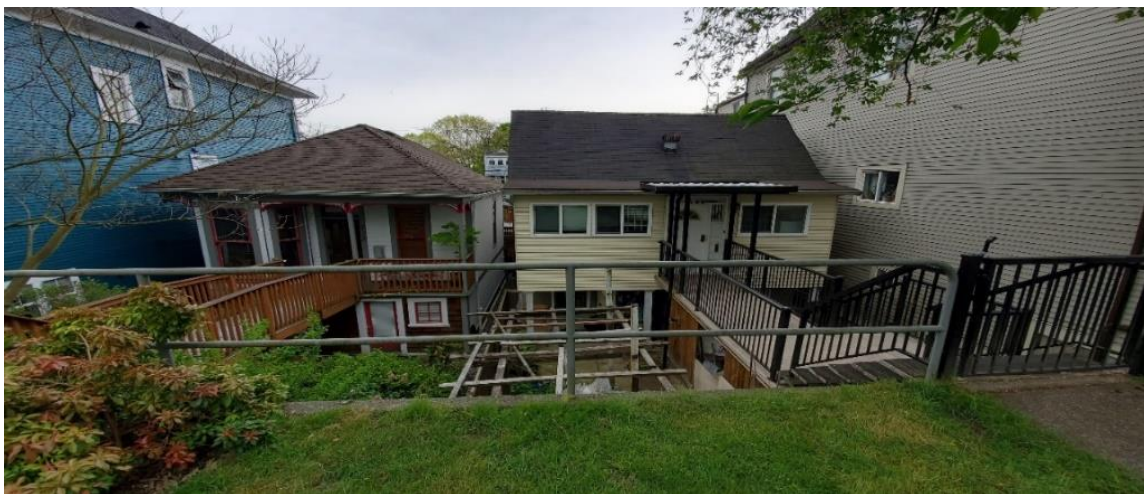
Figure 3. Example of existing grades lower than City building grades
