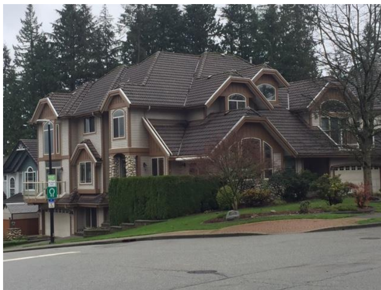
Figure 6. Example of complex roof design
