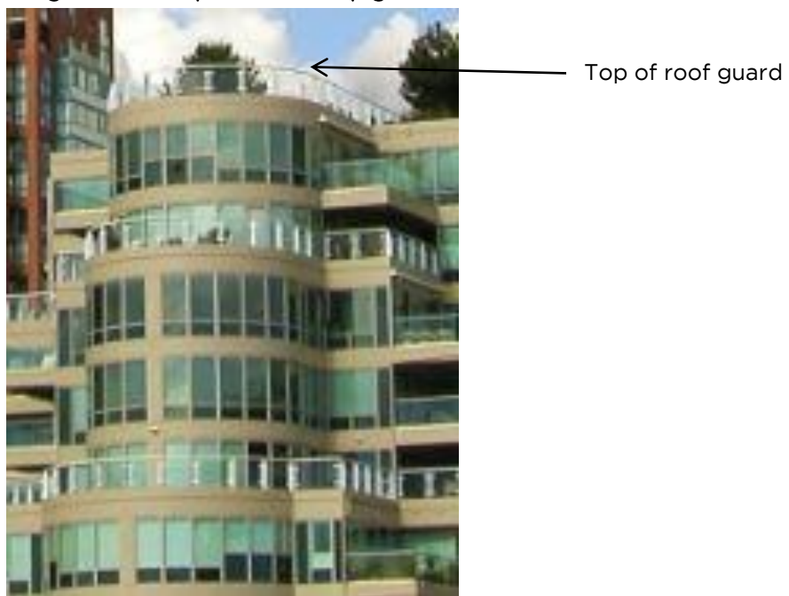
Figure 5. Example of roof-top guard
