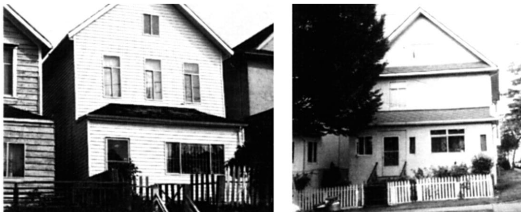
Figure 12. Inappropriate Enclosure
