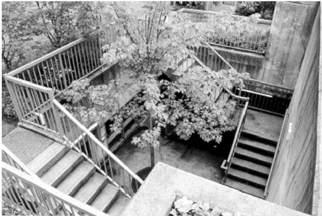
Figure 10. Exits from parking garages can be designed to create a more positive image
