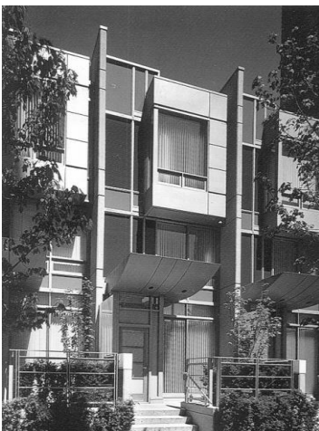
Townhouses: Alberni Street
