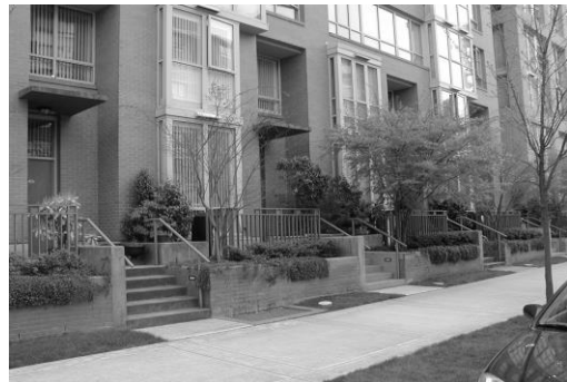
Two-Storey Townhouses Forming Base of Mid-rise Building: Marinaside Crescent
