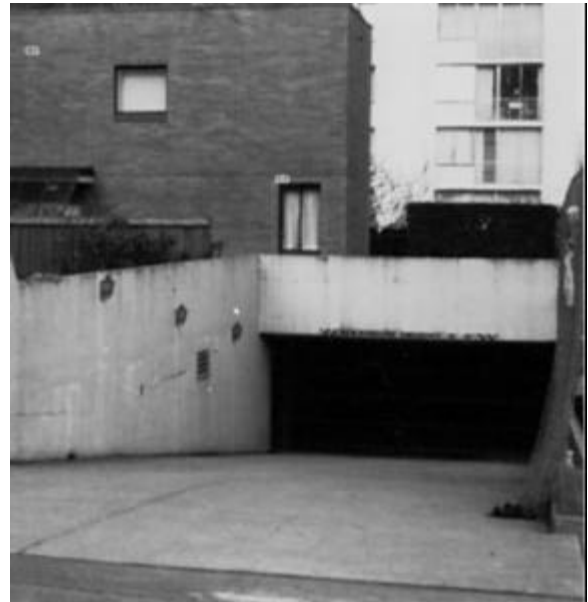
Figure 10. Lack of Quality Treatment of Vehicular and Service Area
