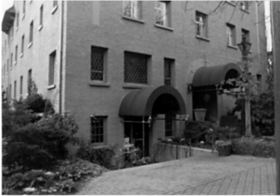
Awnings creating entrance identity and character.
