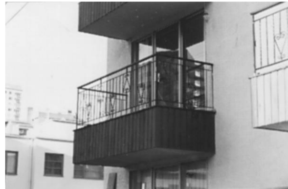
This projecting balcony appears tacked on.
