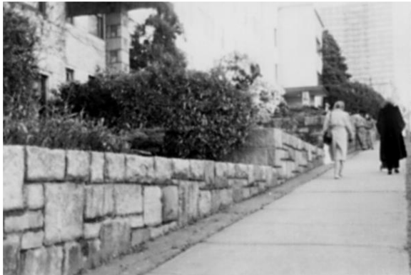
A representative masonry retaining wall.
